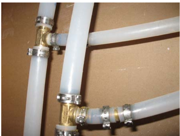
Figure 11: PVC water pipes in a recently built house.
