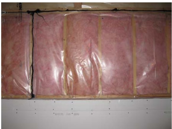
Figure 5: A well insulated basement will help reduce the amount of electricity needed to keep the rest of the house warm.
